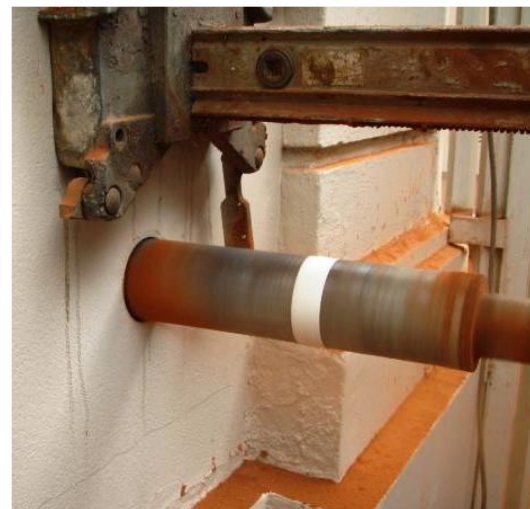
Sampling of wall material for laboratory testing
