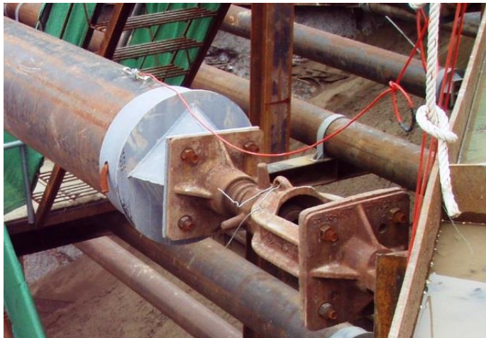
Strain monitoring in lateral support struts
